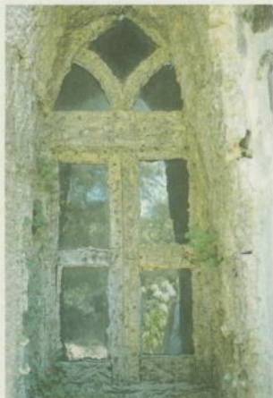
Example of rustic gothic window, with cork frame, presently occupied by the Forestry Government Department
